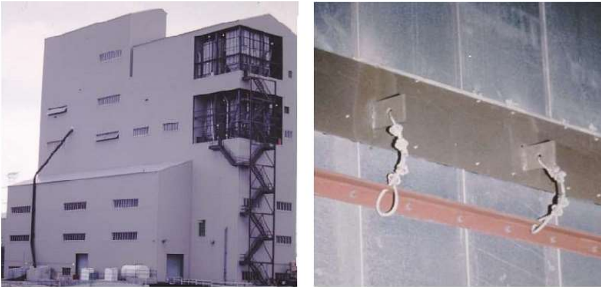
Damage Limiting Construction- Part 2. HCI Systems, Inc.
